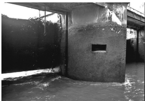
Fig 7. Fish pass on Dłubnia River – view of intake to fish pass through the river channel and the upstream reservoir (photo: G. Gajda)
