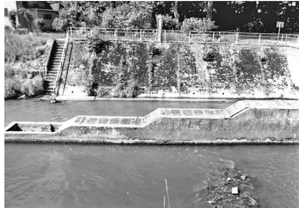
Fig. 3. Fish pass on Dłubnia River – longitudinal profile, side view (photo: A. Radecki-Pawlik)
