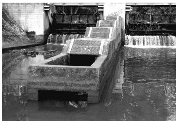
Fig. 5. Fish pass on Dłubnia River – view from downstream after draining the river channel (photo: G. Gajda)
