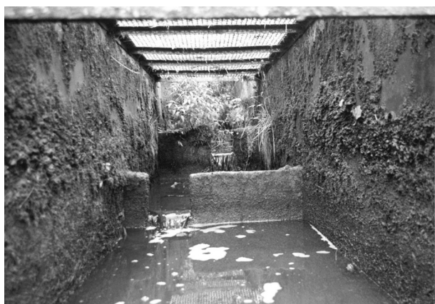
Fig. 6. Fish pass on Dłubnia River – inside view after draining the river channel (photo: G. Gajda)
